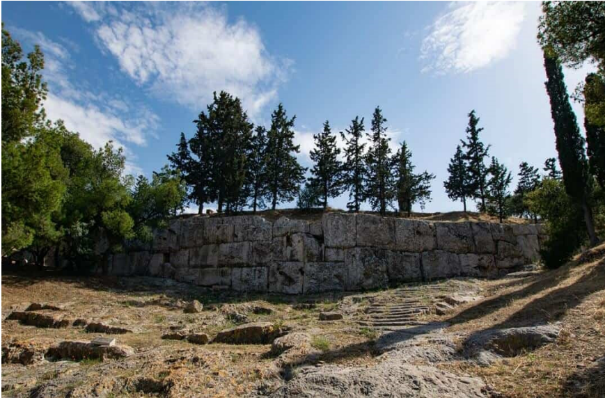
Figure 4c. Remains of the retaining wall built during the third phase of the Pnyx's development. Source: the author.
