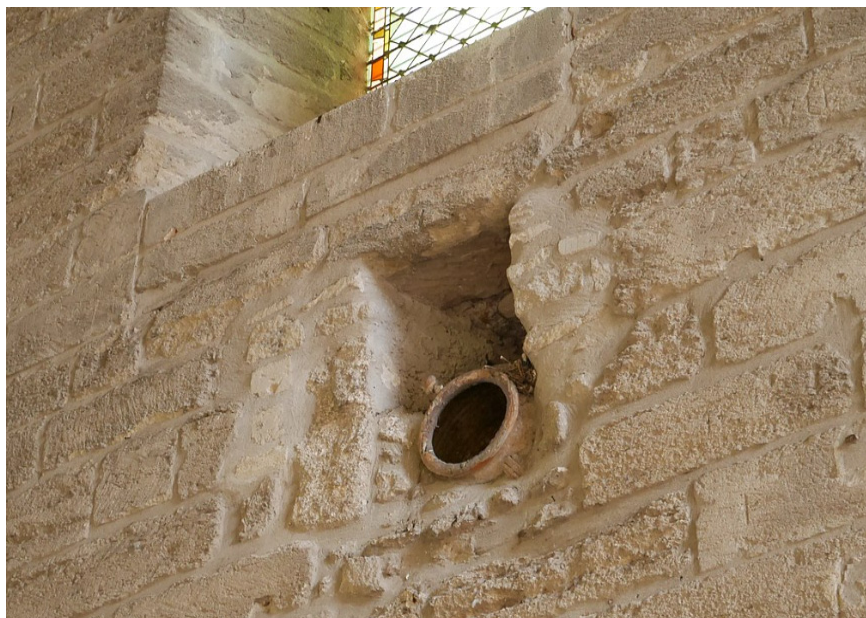
Figure 7. Acoustic pot that is embedded in the wall of the church of the Chartreuse Notre-Dame-du-Val-de-Bénédiction, Villeneuve-lès-Avignon, France. https://en.wikipedia.org/wiki/Acoustic_jar (last visited: 20 February 2023).
